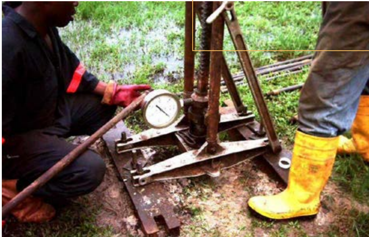
Soil Test to Determine the Most Appropriate Foundation Design for the Project
