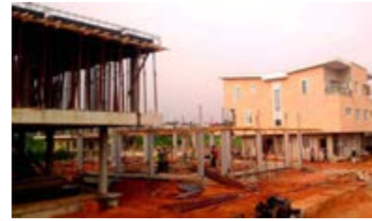
RICHARDS COURT ESTATE Mende, Maryland, Lagos
