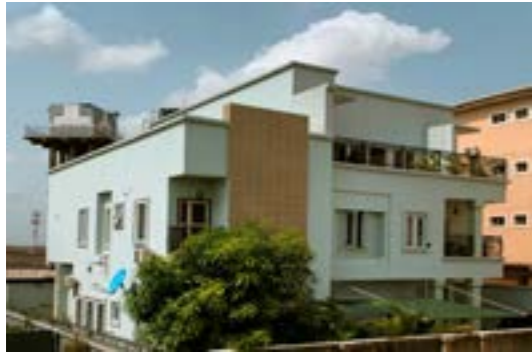
PRIVATE RESIDENCE Anthony Village, Lagos
