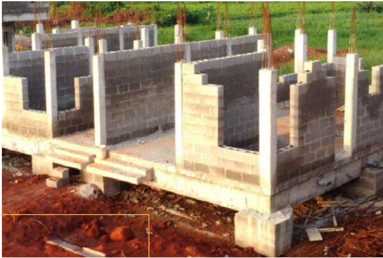
Framed Structure of Pile Caps & Ground Beams
